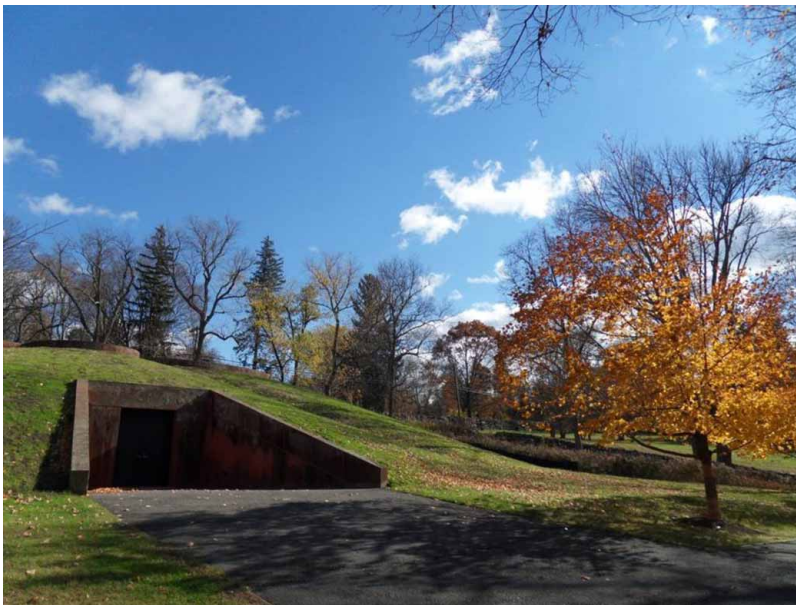
Figure 6. Completed roof replacement and berm restoration. (Mary Kay Judy)
